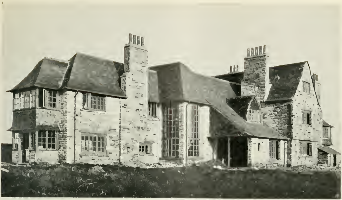
B14 HOUSE AT ST. ANDREWS BELONGING TO CHARLES E. TODD ESQ. IT IS BUILT OF LOCAL STONE AND THE ROOFING IS COMPOSED OF MIXED SLATES FROM EASDALE, CRAIGLEA AND BALLACHULISH
